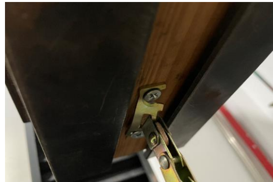
After pulling test
